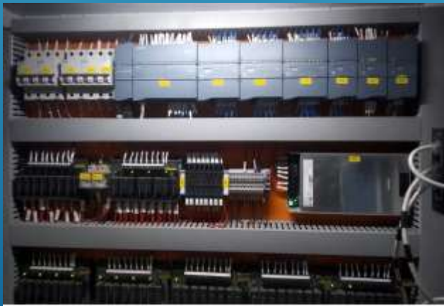
INTERNAL VIEW OF PLC PANEL
